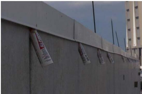
Image of caulk tube used to evict bats from office building. Courtesy of Fly By Night
